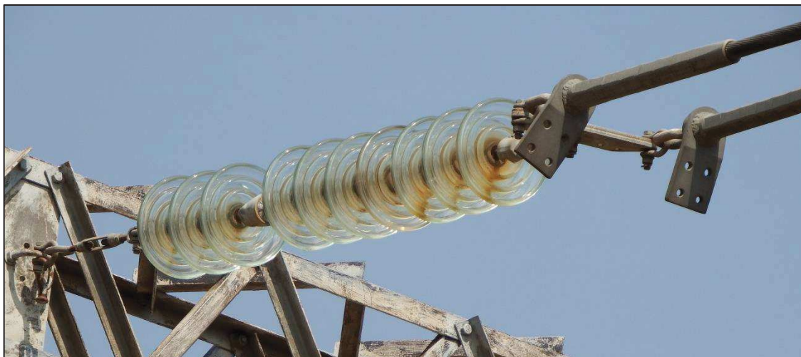
Figure 8: Strain Assembly at Gantry
