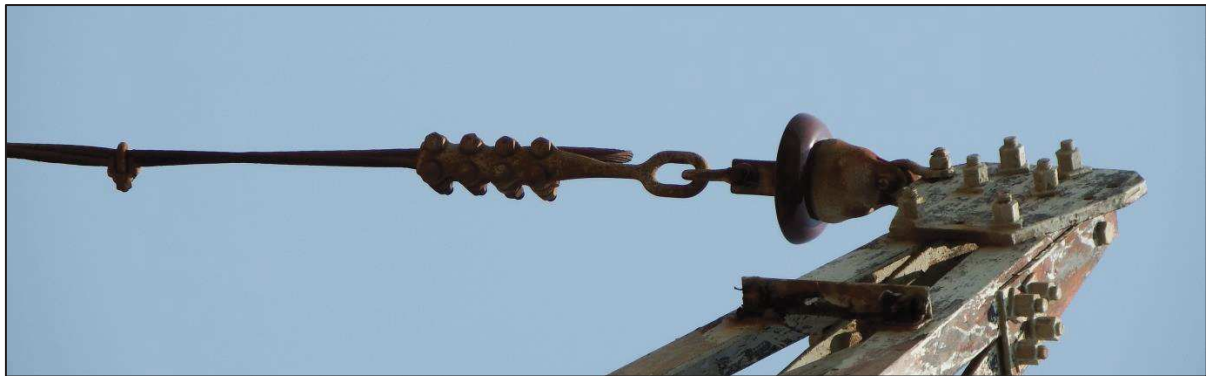
Figure 9: Insulated Earthwire Assembly
